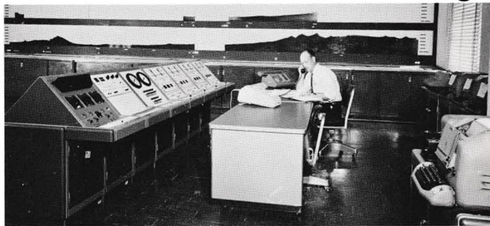
*Figure 5. A typical centralized control station for a pipeline. From this location are monitored such operational details as flow rate, pump pressure and suction, fluid viscosity, and the like. Distant operations can be adjusted in response to changing loads and other variables. Panels in background show profile of terrain which pipeline traverses, and which has important bearing on operating parameters. Centralization is made possible by efficient digital transmission.*
