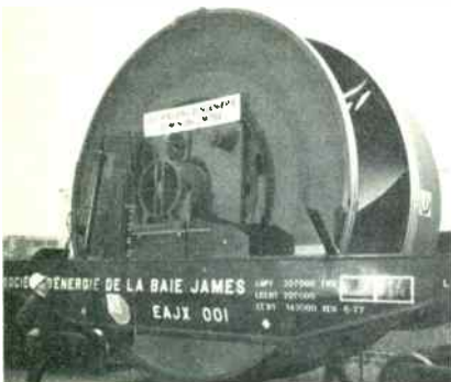
Dominion Engineering employee inspects hydro turbine runner being sent to La Grande 2.
