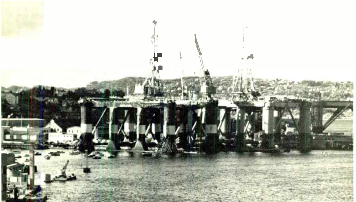
Looking out of scale in the Bergen, Norway harbor, a semi-submersible drill rig, equipped with GE motors and controls, is readied for duty in the hostile North Sea.
