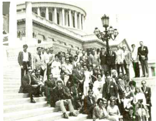
Best Buy suggestion winners from GE's Lighting Systems Business Department saw how their 6,000 lighting luminaires helped reduce the crime rate in Washington, D.C., by 29% and talked with customer John E. Hartley, Assistant Director of D.C.'s Department of Highways and Traffic. ▣
