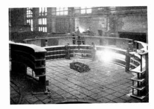
ASSEMBLING THE FRAME OF THE STATIONARY ELEMENT
