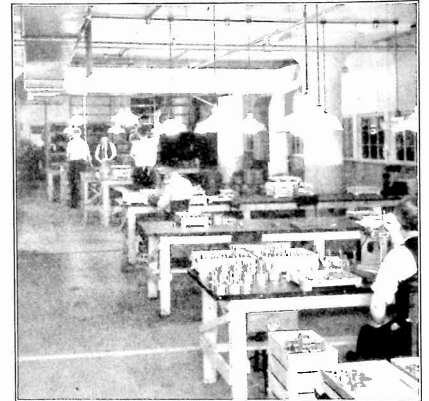
View of a section of the air conditioned testing and measuring department. Conditioned air is brought into this department through the duct which is seen beneath the ceiling.
