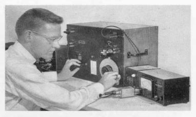
Equipment for 1-mc capacitance measurements. The generator is the Type 1330-A Bridge Oscillator, the bridge the Type 716-CS1 Capacitance Bridge. The null detector (Type 1212-A) is shown at the right. The filter shown is the experimental model; the Type 1212-P2 plugs into the detector in the same way.
