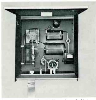
Line Terminating Unit installed in weatherproof cabinet.
