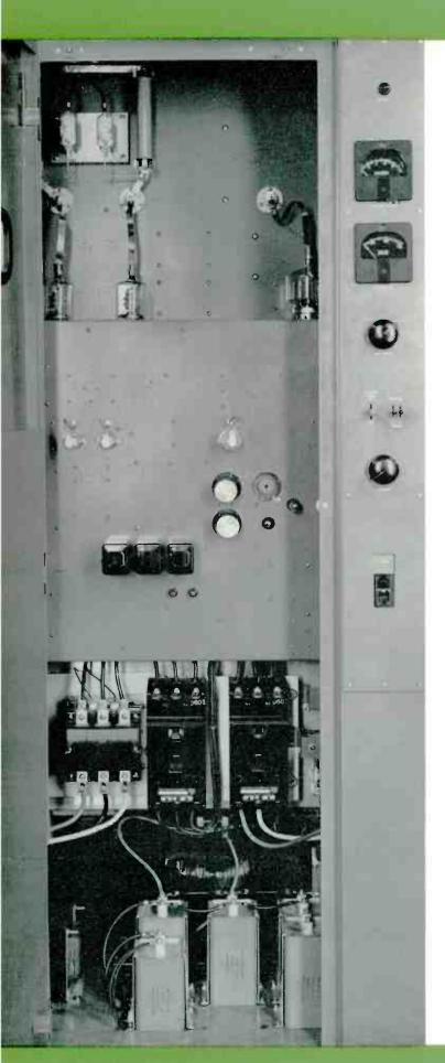
BTA-10U driver including exciter and control panel. Provisions on central panel for third Crystal Oscillator for Conelrad operation is shown.
