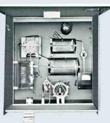
Line Terminating Unit installed in weatherproof cabinet.
