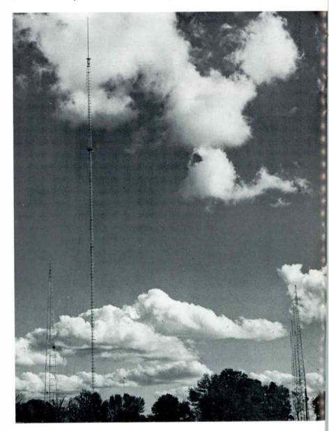
In these multi-tower arrays, methods for sampling the phase and amplitude of the RF voltage in each tower and conveying this sample to the phase measuring equipment located in the transmitter house are required. Accessory phase sampling loops, which are normally mounted on the individual towers, phase sampling lines to connect the loops to the measuring device, and means for isolating the grounded sampling lines where they cross the tower base insulator are also available.
