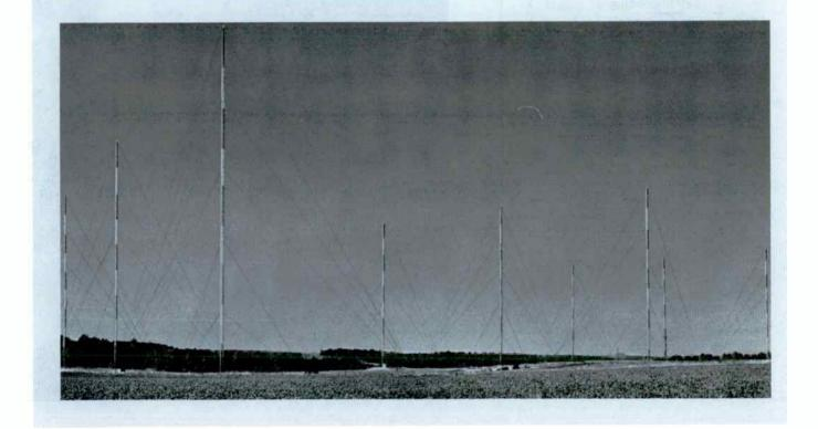
area on all flat surfaces and 20 pounds on round surfaces. This is the equivalent of an actual wind velocity of 86.6 mi/h (139 km/h). Towers with higher windload ratings are, of course, available. Towers are designed in accordance with EIA specifications RS-222B.
