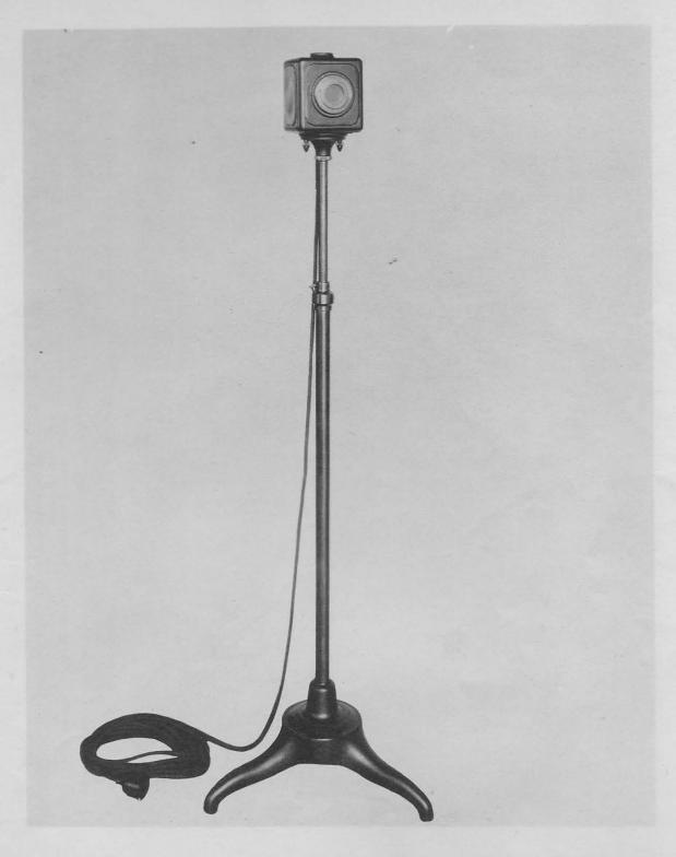
461962 CONDENSER MICROPHONE, AMPLIFIER, AND PROGRAM STAND, TYPE 4-AA, DL-7550657G-2. WALL RECEPTACLE NOT SHOWN.
