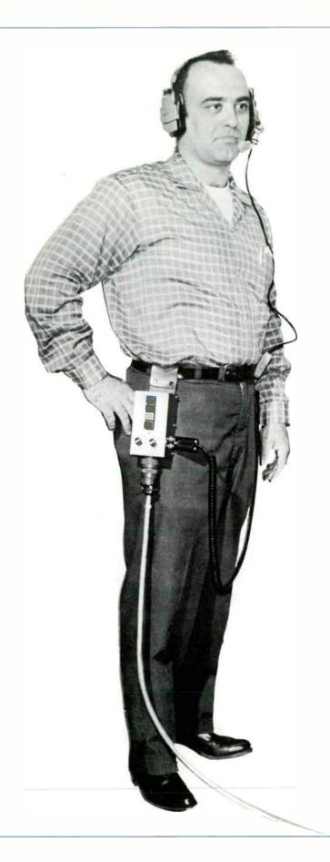
Unique "belt box" station for studio floormen. The box hangs on his trousers belt and connects him with the intercom system without restricting mobility. Four pushbuttons give him two-way communication with as many stations on the intercom system.
