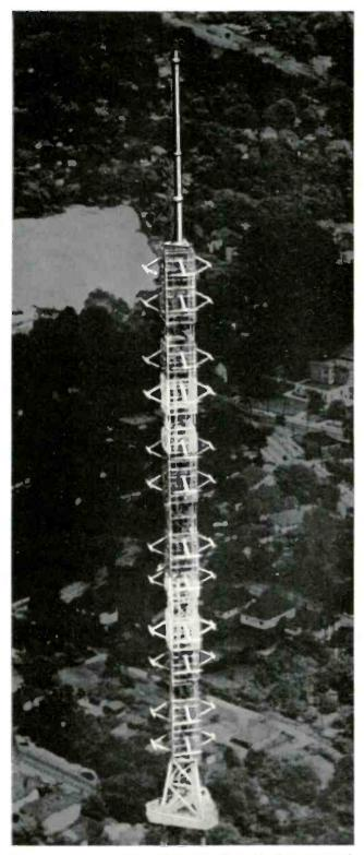
Supergain Antenna at WSB, Atlanta, Ga. Since this photo was made, the antenna has been changed from a 12-section to a 14-section type.
