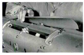
View illustrating how polyethylene protective covers are placed over all slots to protect the inside harness.
