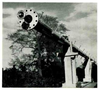
Bottom view of an RCA UHF Pylon Antenna showing the mounting flange and the transmission line connection.
