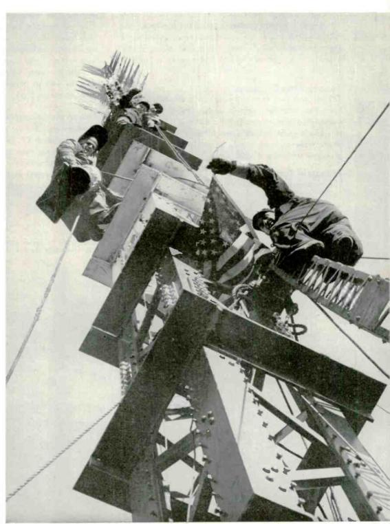
Photo showing a closeup of the "multiple-use" TV antenna supporting tower located atop the Foshay Building, Minneapolis, Minn. The seven diaphragms on lower portion are for strengthening and permit supergain elements to be mounted in between them.
