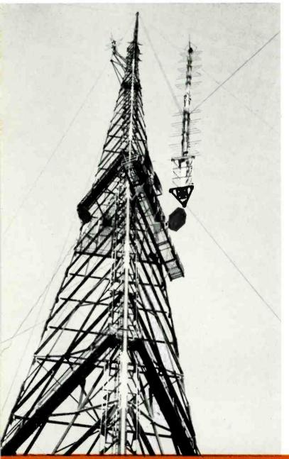
of the radiator. The line feeds the center of the radiator, at low impedance, so that ice formation has little or no detrimental effect. Such ice formation can be alleviated by the use of sleet melting resistors which are available as accessories.
