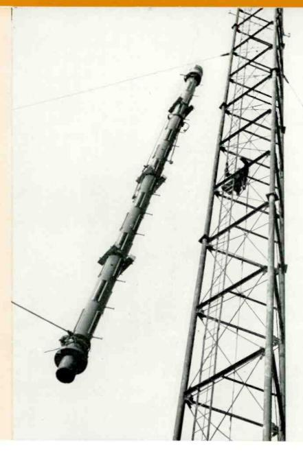
View taken at the 300-foot level of WKNB-TV's (New Britain, Connecticut) tower where the RCA UHF Pylon is shown "on-the-way-up". Note that erectors easily handle the RCA antenna as a single unit, thereby reducing precious installation time.
