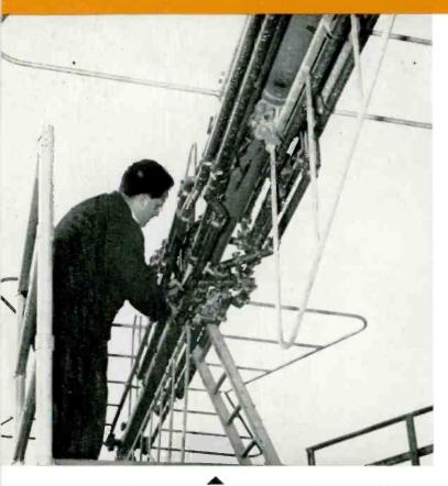
Closeup photo showing the construction of a special copper feedline diess for a custom designed RCA Superturnstile Antenna.
