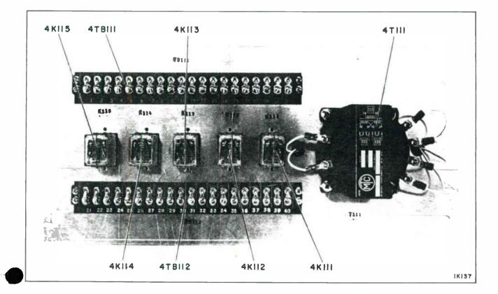
Figure 17. Remote Control Relay Panel MI-561354 (Prefix 4)
