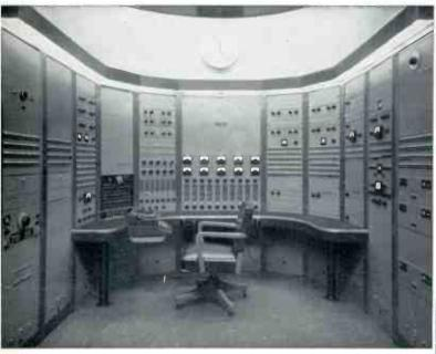
WNEW, New York. This master control installation—in WNEW's seven-studio lineup—is flanked on each side by five deluxe audio equipment racks. It has complete facilities for control and preset switching of seven studios to ten outgoing lines . . . and for feeding cues from any channel to any studio.
