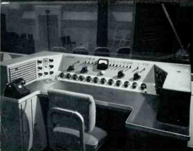
WJAC, Johnstown, Pennsylvania. In this speech input layout, custom-built matching-end consoles contain auxiliary switches and controls. They are used in conjunction with a standard 76-series consolette to provide increased flexibility and convenience.
