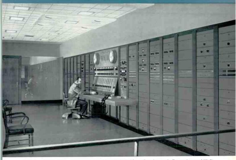
WBAP, Fort Worth. The master control installation pictured here includes 16 deluxe audio equipment racks. These are just part of WBAP's modern six-studio layout. The master control installation features an "In-Line" design for handling 16 inputs and 10 outgoing channels.
