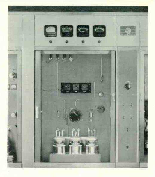
Front View of the R-F Output or Power Amplifier Cabinet showing the arrangement of RCA-5762\* Tubes, Controls and Components. Other circuit components and wiring are accessible by means of the rear sliding doors.
