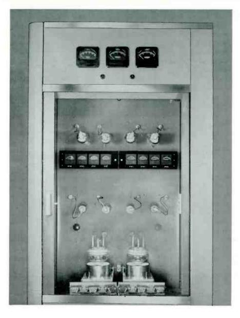
Closeup View of the Audio and Modulator Cabinet showing the mechanical and electrical arrangement of major components. Long-life RCA 828's, 807's, 813's and RCA 5762's are employed in these stages. Bi-level modulation reduces distortion and increases fidelity to a new high in the BTA-5H.
