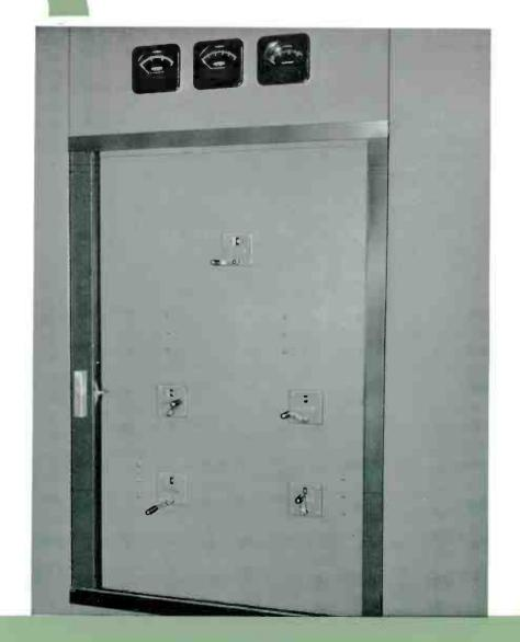
Phasing equipment installed at Radio Station KSOO is housed in the new type horizontal sliding door cabinets. Cabinet at right contains the power and current dividing networks for each tower and day-night pattern-change relay.
