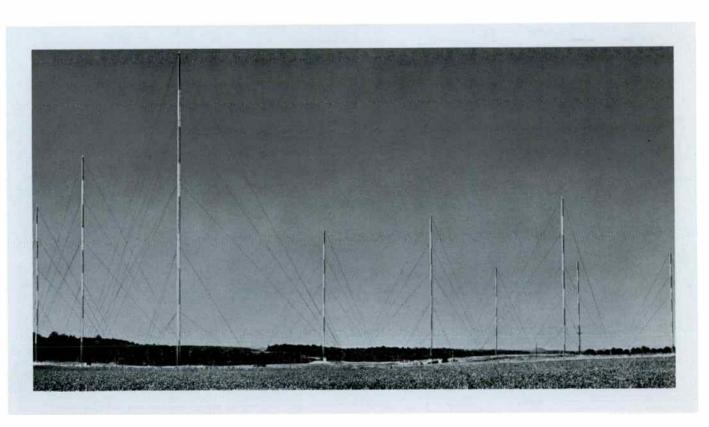
area on all flat surfaces and 20 pounds on round surfaces. This is the equivalent of an actual wind velocity of 86.6 mi/h (139 km/h). Towers with higher windload ratings are, of course, available. Towers are designed in accordance with EIA specifications RS-222B.
