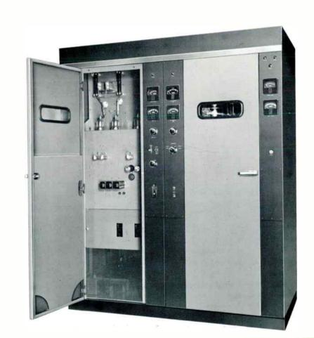
IPA and modulator driver stages of the BTA-5TI can be seen at top of open cabinet. The exciter is at the center of the cabinet, and control equipment is placed just below the exciter
