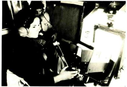
With the port-side panel removed, the TV camera has a virtually unobstructed view. Each Goodyear blimp contains a Fernseh KCT-40 camera system with Terracom GCN-6.2 GHz microwave and Schneider 30 X 12.5 lens. (*Photo courtesy of Goodyear Tire & Rubber Co.*, Airship Operations)
