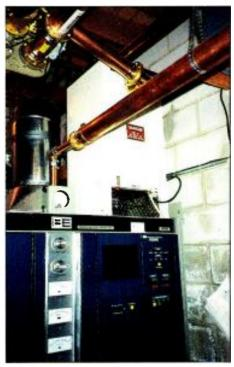
Reject load above KBSU's Broadcast Electronics FM-10A transmitter.
