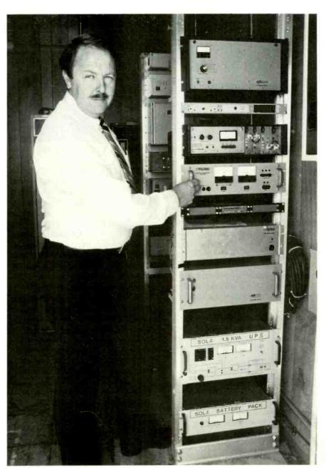
Hutchinson points out the Sola 1.5 kVA UPS installed at the relay site.
