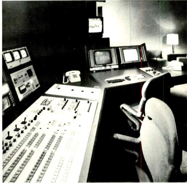
Ultimately, systems will develop that will allow the application of all of Editel's video editing power to be applied to film. Editel's main editing suite includes the Mach One editor, Grass Valley 1600 7H switcher with E-MEM, and Vital Squeezezoom digital video effects
