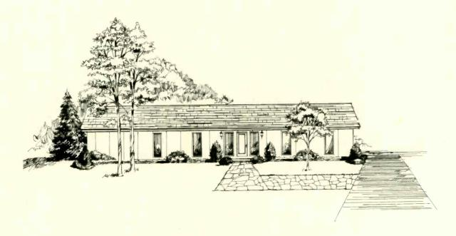
One of exteriors available with standard Grinnan prefabricated broadcast station building is shown in the drawing above. The exterior walls can be lapped siding, brick veneer, brick, stucco, plywood panels, or others. The roof can be gabled (as shown) or flat, with one side of the roof covered with acrylic plastic if solar heating is chosen
