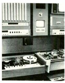
Two views of AHA's studio setup showing IVC one-inch recorders (with TRI editor) and camera control racks.
