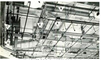
(A) LOWER GRID (B) UPPER GRID (C) CYCLORAMA & DRAPERY TRACKS (D) FLOOR OF PERIPHERAL CATWALK (E) CYCLORAMA LIGHTING OUTLETS (3 color)
