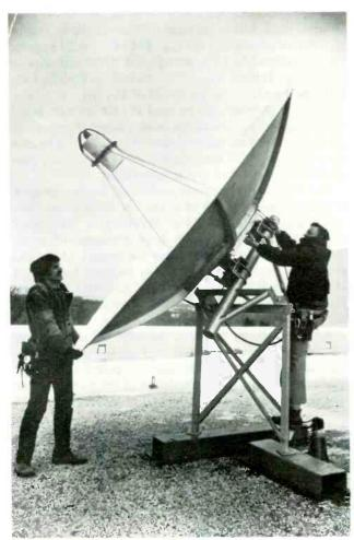
Antenna for Western Union receive-only earth terminal is this 10-foot dish, being set on roof of WU headquarters in New Jersey. Small size and weight of antenna allows installation on roof of radio studio or nearby.
