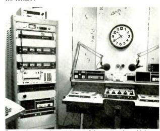
Production room is modular pre-fab construction which can be moved. Walls include large glass panels.
