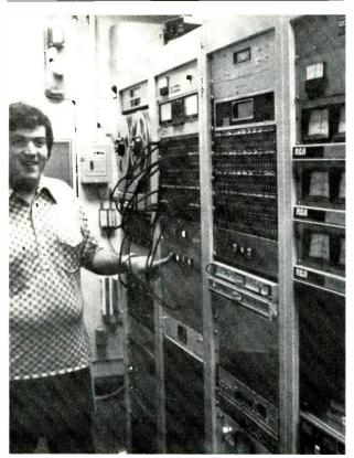
Patch panels, remote transmitter controls, logging recorders at WQXI are located in a separate engineering equipment room.
