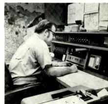
Core of news center is the Dispatch Center. At right is specially built Motorola console. At left are incoming microwave feeds.
