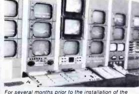
For several months prior to the installation of the BCS business system, the schedule prepared by traffic was typed into the CDL system using CDL terminals in traffic. Last minute changes are handled by the keyboard in master control (lower left).
