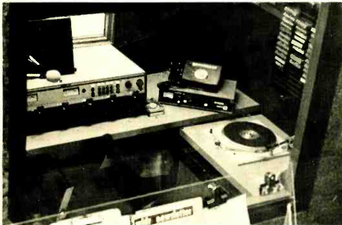
Production Control Room (seen from FM Master Control)
