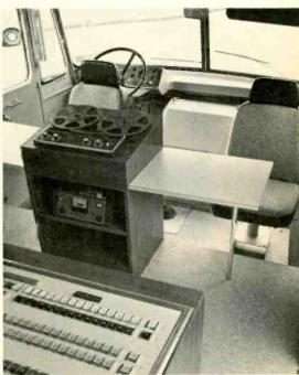
Interior shot of Mobile Television van used for special events broadcasting shows Tapecaster cart machine underneath a reel-to-reel machine. Van also carries three Ampex BC-230B color cameras.
