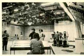
Interior of Studio A shows lighting control board in use. Three Ampex BC-230B color cameras are in use in the background. The control room is at the right behind glass.
