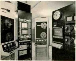
Fig. 6—Some of originating equipment in master control is Sony MV-10000 helical VTR, (left and center right), Datatron editor, TMI time base correctors, Tektronix monitoring and test units.
