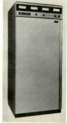
World's first 1 kW solid state transmitter.
