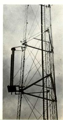
Standby antenna is twentyfoot section added to one leg of WSBA tower. It's easily adjustable in field for proper pattern.
