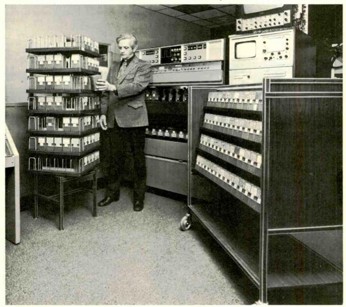
Illustrated is 7-tier Carrousel (140 cartridge capacity) on a CS-16 Ball Bearing Base, and VTS 16-18 Stand; and CTC-128 Transport Cart (capacity 128 cartridges).
