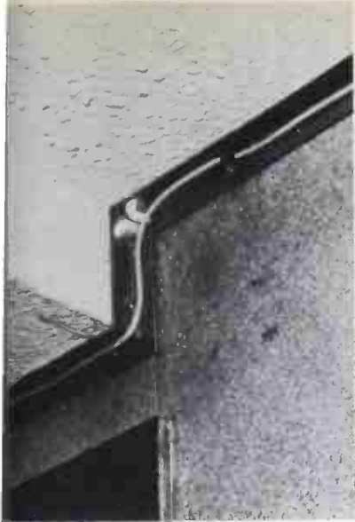
Molding channel is installed inside public hallways. A molding strip snaps into place concealing cable.
