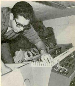
There is easy access to the control console at KVEC. Consulting engineer Glenn Daly checks wiring at the console rear. All audio cables run through plastic Panduit to a slide-out rack in the back of the console, or to patch panels in various inbuilt racks.
