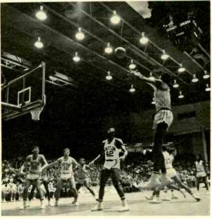
Good top and side lighting is maintained on players, floor, and baskets at the U of D Arena by a total of 62 mercury 1000-watt lamps and 30 Quartzline 1500-watt installations.
