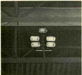
Mounted 60 ft. outside the court sideline, and 60 ft. above the playing floor, three 5-lamp groupings of 1500-watt Quartzline lamps provide illumination on vertical surfaces on the playing floor, to assure good TV pickup from both sides of the court. Catwalk behind lamps permits easy maintenance.
