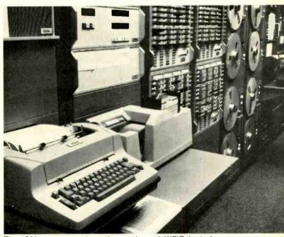
The IGM program automation system at WFIR includes a logging typewriter (foreground) and card reader just past it. Next are two racks of Instacarts and two more of Scully reel-to-reel decks. Finally, a Moseley automatic logger and transmitter remote controls.
