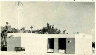
Compact, efficient KANW studio-transmitter building is a double hexagon, minimizes parallel walls in studio. Tower is behind building, adjacent to transmitter room.
