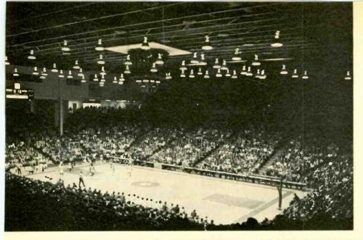
At the University of Dayton Arena, overall court lighting is ample and even. A row of mercury lamps 40 ft. above and 15 ft. outside each sideline assures coverage there and reduces contrast between the first few rows of seats and the court.
