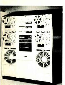
The RCA DAP-5000 digital automatic programmer (center dark panel) is surrounded by carousels, open-reel tape, and single-play cart machines.
