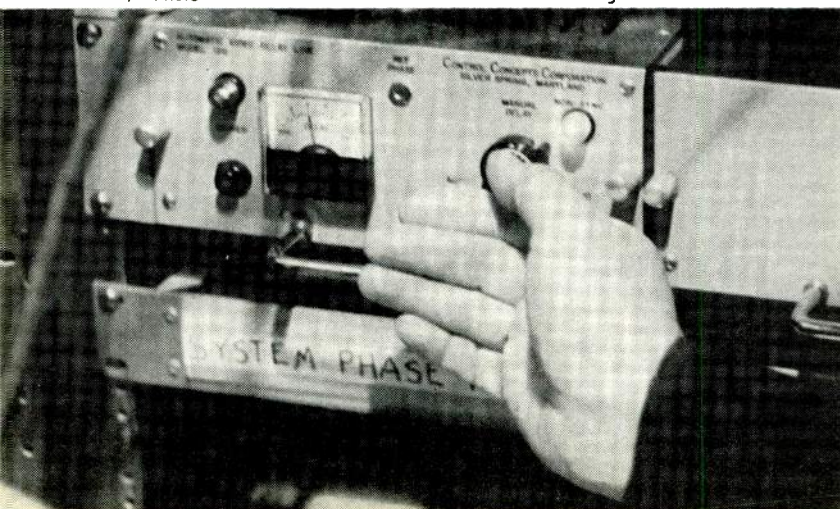
Automatic delay line by Control Concepts Corp., as installed in ABC Network's New York switching control.
