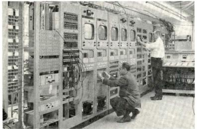
Television coverage of this year's Olympics near Mexico City is being distributed to worldwide broadcast networks and their viewers from this switching complex, manufactured at RCA's Camden, N.J. plant. The \$750,000 system, one of the largest ever built, is capable of handling up to 24 incoming program signals simultaneously and distributing them on 12 outgoing lines.
