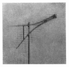
30' parabola developed by Hosken. Firm is now installing 100' unit for Pittsfield (Mass.) Cable TV, mainly to receive New York signals originating 125 miles away. Hosken recommends use in pairs to eliminate co-channel and adjacent-channel interference. New "Exponential Curved Antenna" developed by Hosken is reported to have high gain, excellent rear rejection, and wide-band characteristics necessary for color. Reception quality is said to be superior to that achieved with yagi design.
