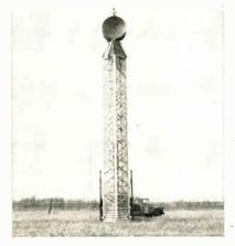
Stacked sections are pulled upright by tower guy wire. Rising sections pull remaining guys into place. No extra equipment required. No scaling of tower necessary. All erecting is controlled from ground level. Easily erected by five man crew.
