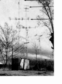
Head-end site of Placerville, Cal., system. Five-element channel 4 yagi (top arrow). Four 10-element yagis stacked in "box array" configuration for increased gain (center). Four 10-element yagis stacked horizontally to reduce Channel 9 co-channel interference by attaining a sharper frontal lobe (bottom).
