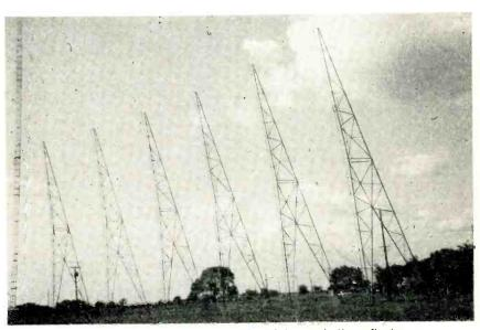
Fig. 5. Completed 150-ft. long by 80-ft. high parabolic reflector.
