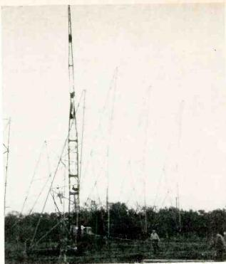
Fig. 9. A crane is used to lift the top section in place after the first section is anchored to the concrete base.
