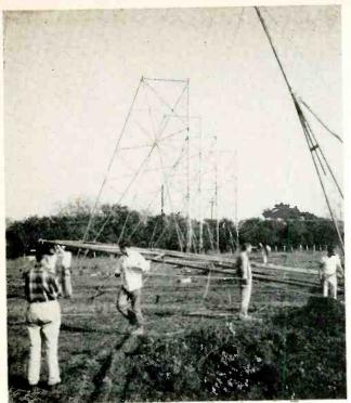
Fig. 8. During construction, the first 40' of each A-frame is erected, then the top section is placed, usually with the aid of a crane.
