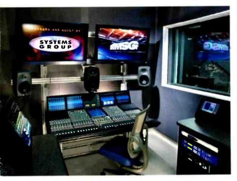
The "multipurpose" room at MSG Media's facility, in New York, houses the Solid State Logic C100 HDS console. The board's primary use is for live audio mix, voice-over and SAP.
