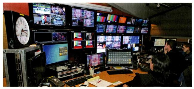
Blackmagic Design's Broadcast Videohub routers come with SDI reclocking features, allowing ProShow to connect to longdistance equipment, as well as redundant power supplies and power fail protection.
