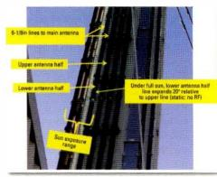
Figure 11. Transmission line configuration on tower
