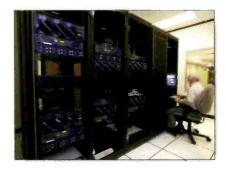
nected directly to the central storage infrastructure through a high-speed, high-availability 2Gb Fibre Channel redundant SAN fabric.
