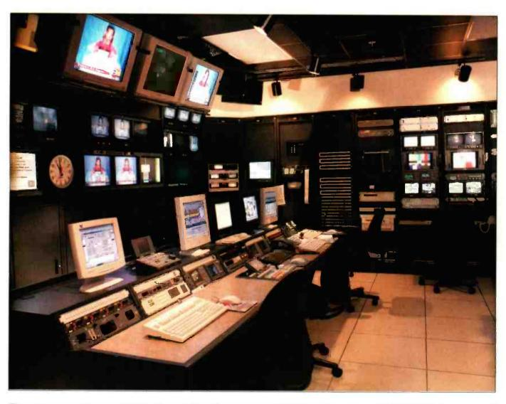
The master control room at WWSB Channel 40 utilizes Sundance Digital's Intellisat to control the Omneon networked content server system for satellite ingest. Also displayed are the Sundance Fastbreak on-air and prep stations.
