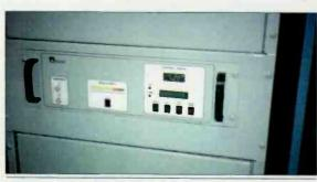
Digital FM exciters like the Nautel NE-50 are typically available with either analog or AES/EBU digital audio inputs.
