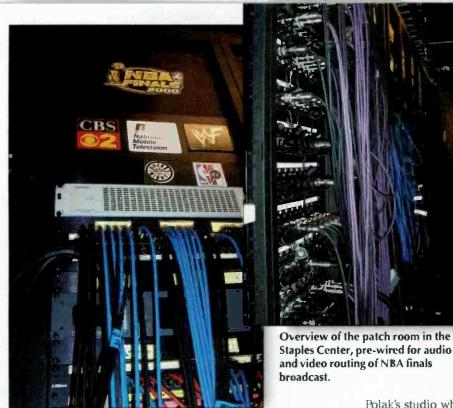
Audio patch panels in patch room of the Staples Center, wired for a radio broadcast of the WNBA Sparks.
