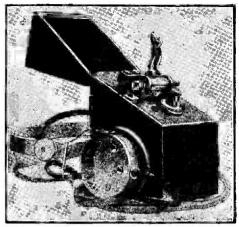
Fig. 11.—Three-quarter View of Variometer Crystal Set.
