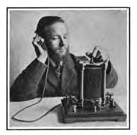
FIG. 97.—Bellini-Tosi radio-goniometer for directive wireless telegraphy.
