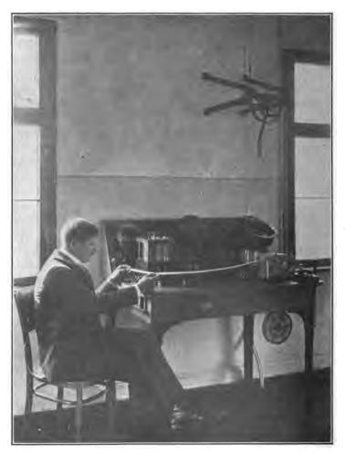
FIG. 119.—The receiving apparatus of the station at Nauen. The message is being printed on tape by a recording device.
