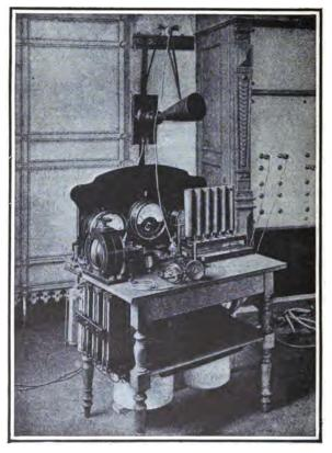
FIG. 147.—Poulsen wireless telephone equipment.
