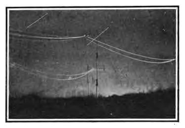
FIG. 149.—Showing the brush discharge from a Marconi transatlantic aerial at night.
