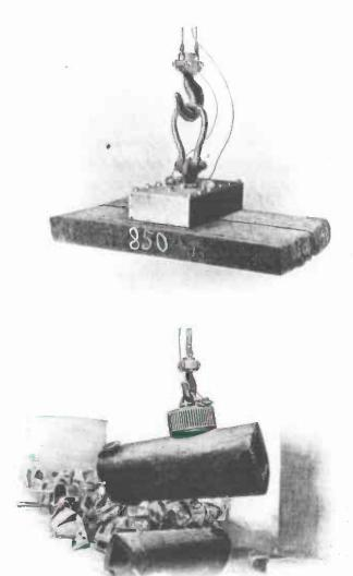
By permission, from "Solenoids," by C. R. Underhill. LIFTING-MAGNETS OF THE TYPE KNOWN AS PLATE, BILLET, AND INGOT MAGNETS.
