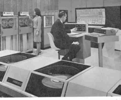
Computer installation with disk packs in foreground and tape drives at left.
