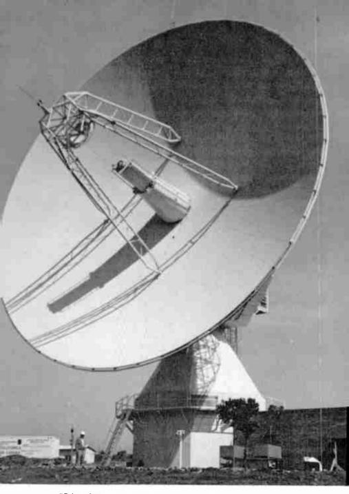
85-foot-diameter antenna at ground terminal in Buitrago, Spain was designed and built by ITT to serve as communications center for intercontinental message traffic.
