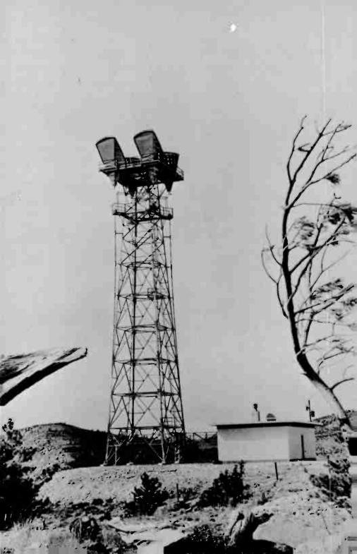
to being plowed up or otherwise damaged, as are cables and wires. Transmission by microwave is generally immune to such atmospheric problems as static and lightning.
