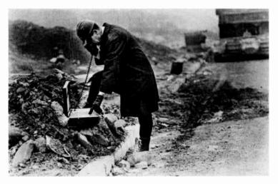
A portable telephone at a construction site saves installation of temporary phone lines.
