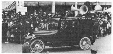
In 1925 KGW, Portland, Oregon, used this car to broadcast to people on the streets through loudspeakers the KGW signal picked up by a receiver in the truck. Before long some enterprising individual reversed the process, and mobile broadcasts were made from transmitters mounted in practically all kinds of vehicles.
