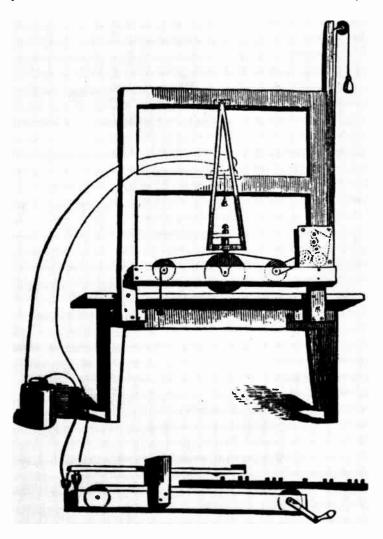
Left The original drawing on which Morse based his patent. The key at the bottom taps out the code, which is marked on the paper roll by a pen, held in the iron triangle, moved by an electromagnet.
