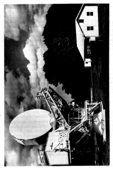
Fig. 3—Crawford Hill main receiving facility showing 7-meter diameter antenna and control building.
